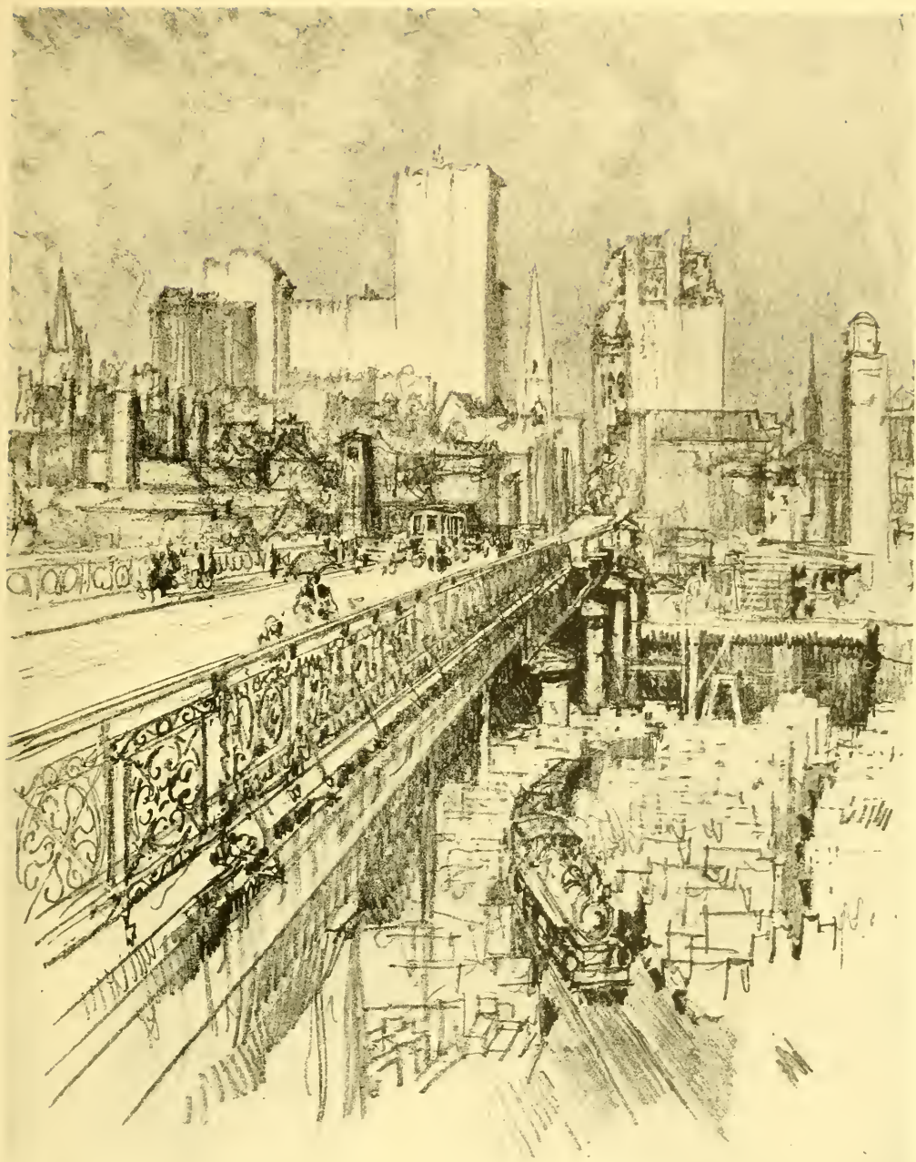
CHESTNUT STREET BRIDGE
